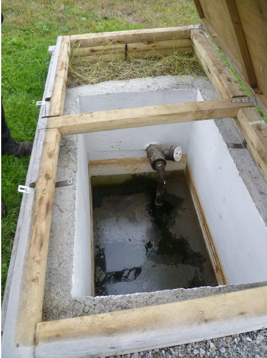
Repaired oil interceptor
