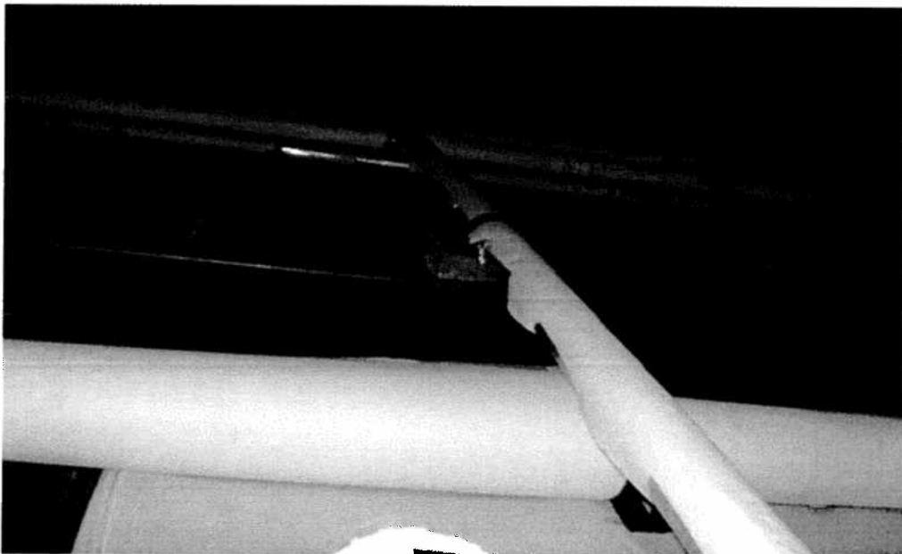
Fig 4.1 – Water lines above suspended ceiling.
