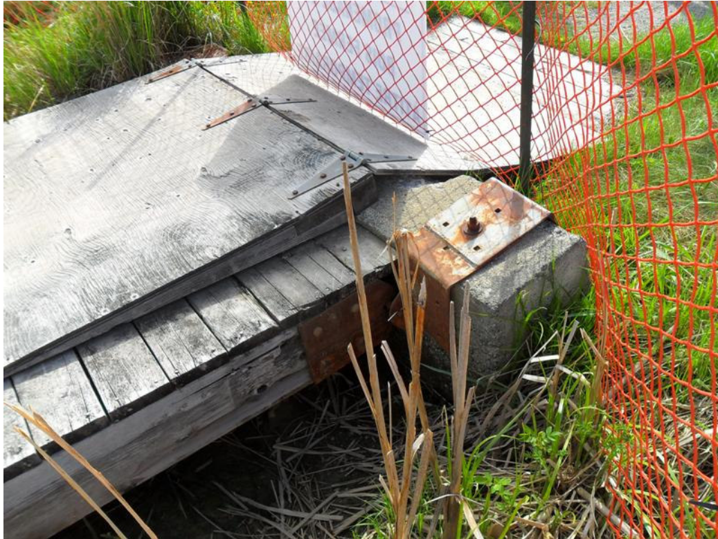
Photo 9 – Start of boardwalk and connection to abutment.
