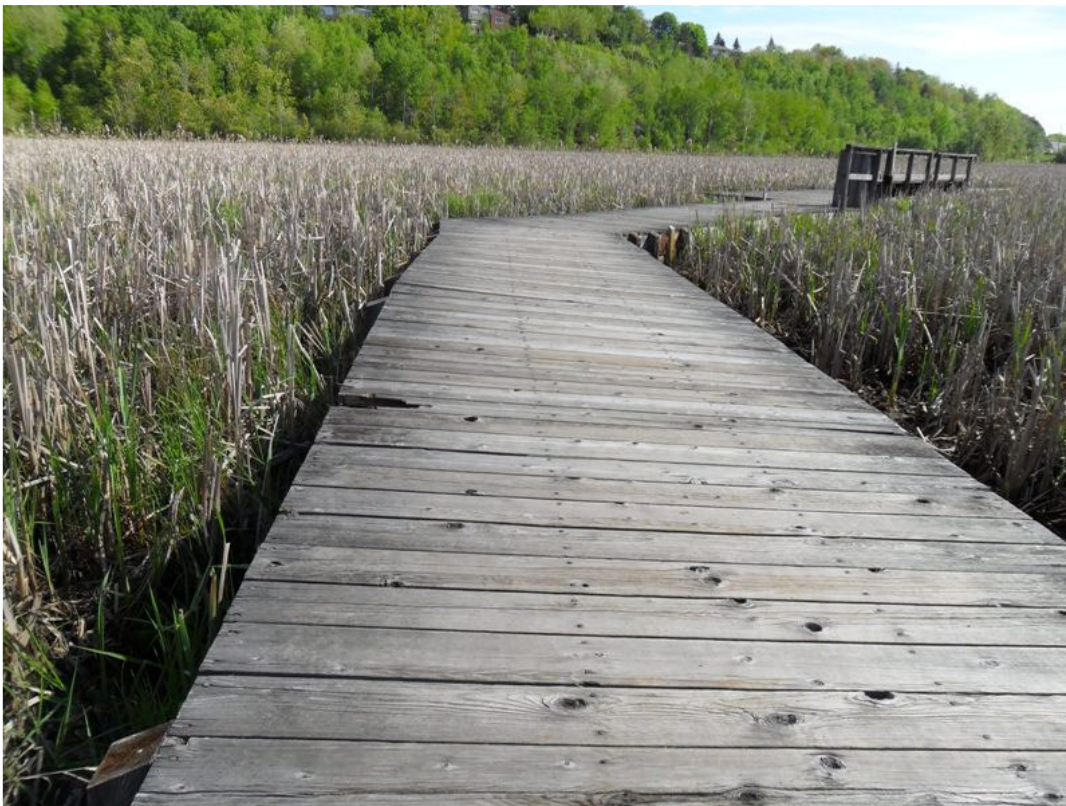
Photo 2 – Boardwalk sloping to side.
