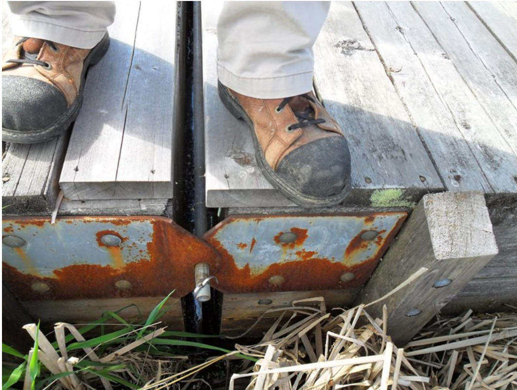
Photo 5 – Panel connection showing mild corrosion.
