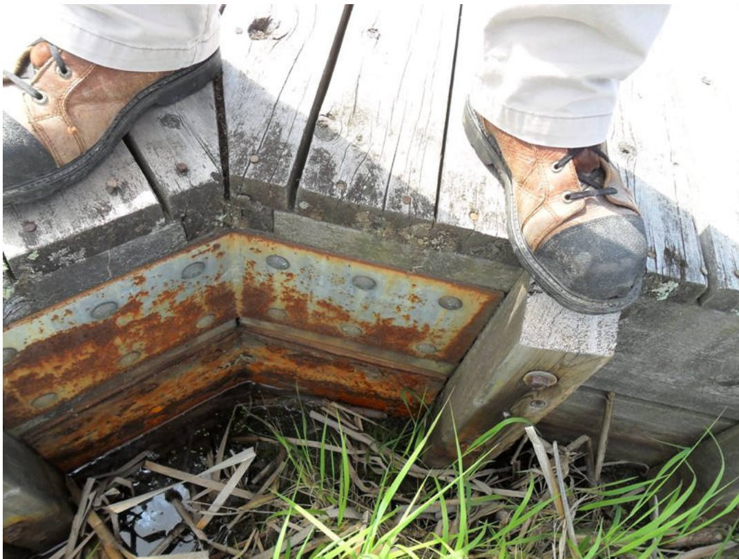
Photo 6 – Metal connections corroded below water line.
