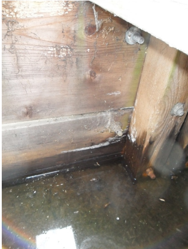
Photo 3 – Boardwalk sub-structure – rot and corrosion below water line.
