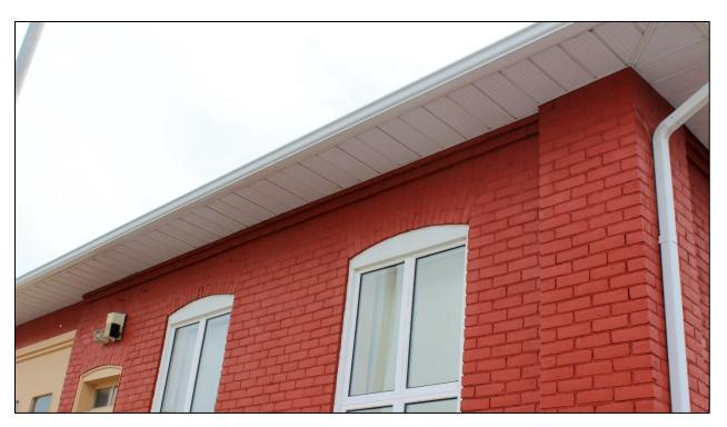
Figure 29: Detail of the northern elevation windows with brick voussoirs (Source: ML, 2020).
