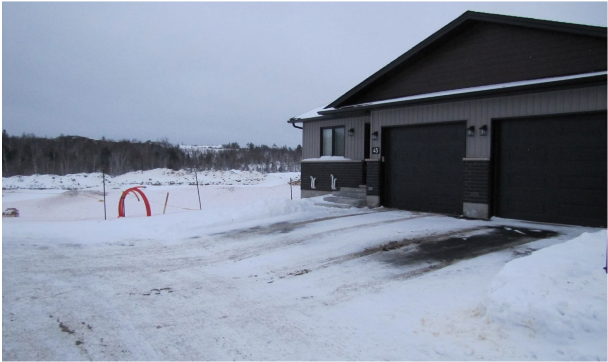
Photo 2. Subject lands, south of 250 Billiard's Way, facing south, showing unit #45 and #44 in the foreground (labelled as #44 and #43 on the concept plan). Photo taken January 22 , 2024. CGS File 751-6/23-18.
