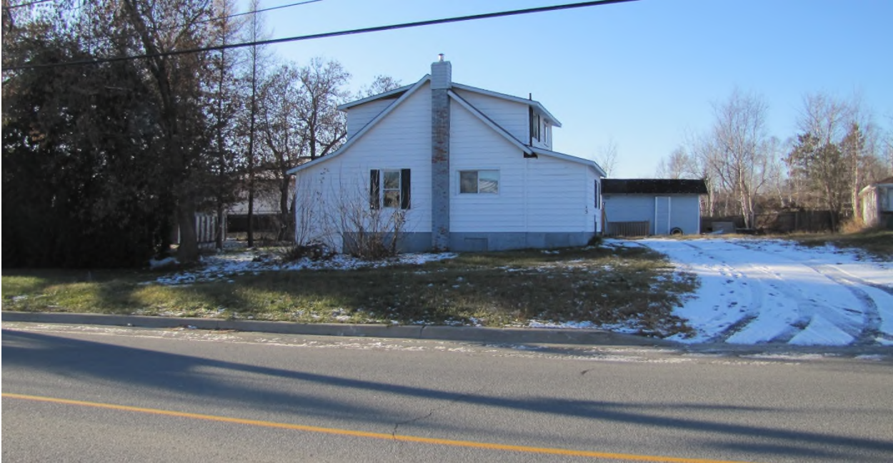
Photo 1. Subject lands, 15 Levesque Street, facing west. Photo taken November 24, 2023. CGS File 751-6/23-19.
