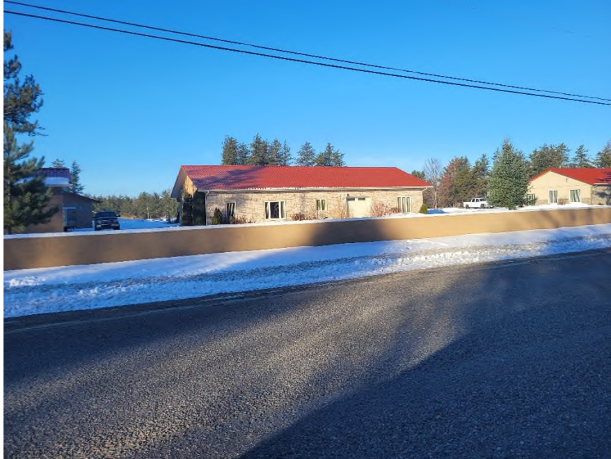
Photo 1: 3891 Hydro Road, Hanmer
