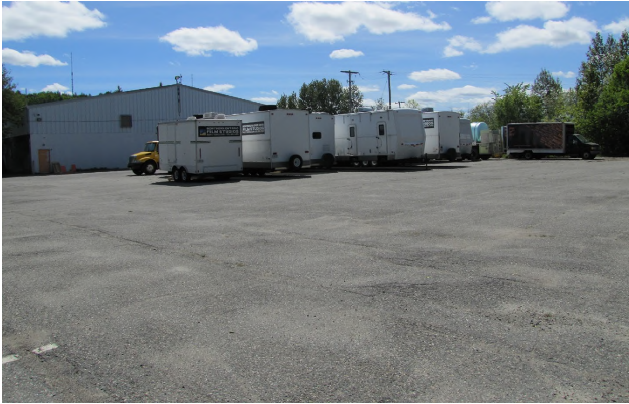
Photo 4. Subject lands, 828 Beatrice, facing southwest, showing the existing arena building and parking area. Photo taken May 24, 2024. CGS File 751-6/24-09.
