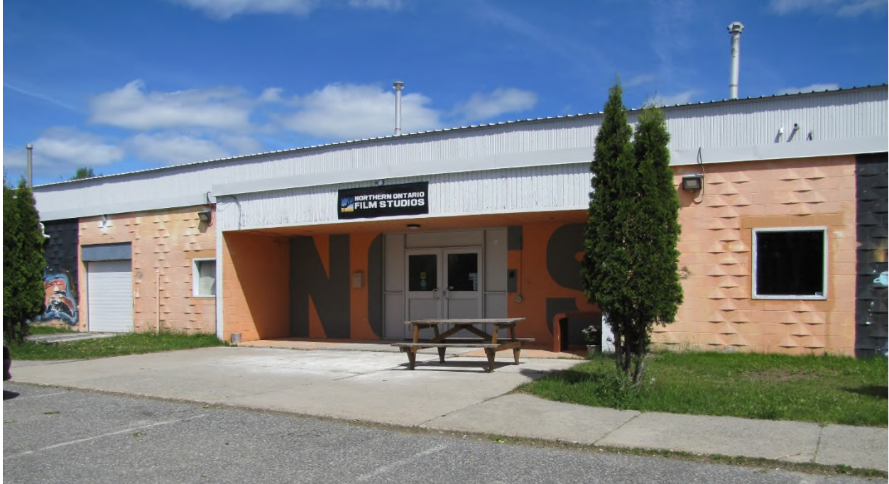
Photo 3. Subject lands, 828 Beatrice, facing east, showing the 'main entrance' to the existing arena building. Photo taken May 24, 2024. CGS File 751-6/24-09.
