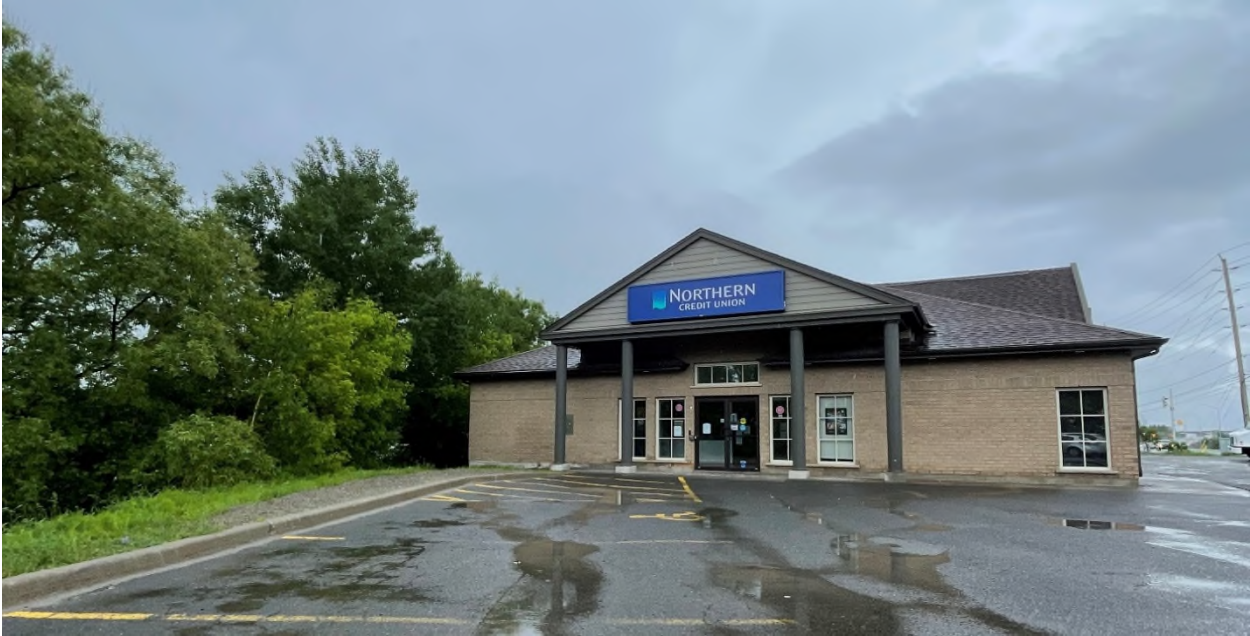
Photo 3. Subject lands, 2380 Long Lake Road, Sudbury. Photo taken from the north facing south on June 6 th , 2024. CGS file 751-6/24-03.
