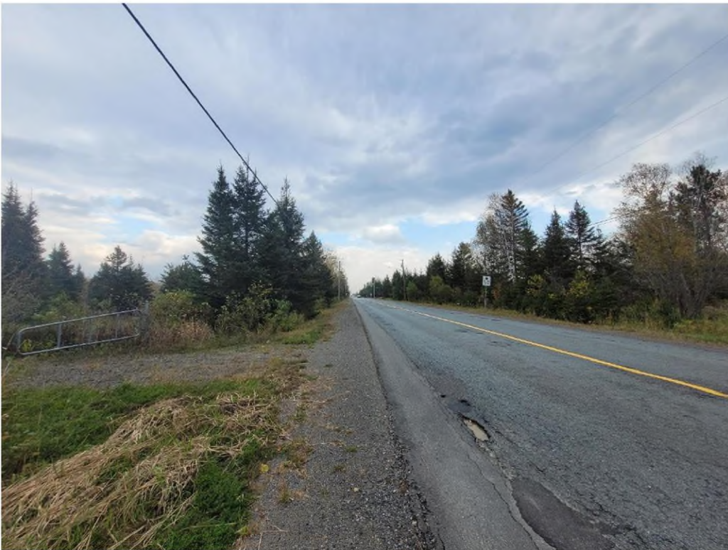
Photo 6: 0 Dominion Drive, Hanmer. View of the Dominion Drive looking west with the subject parcel to the left File 751-7/24-07 & 701-7/24-01 Photography: October 6, 2024
