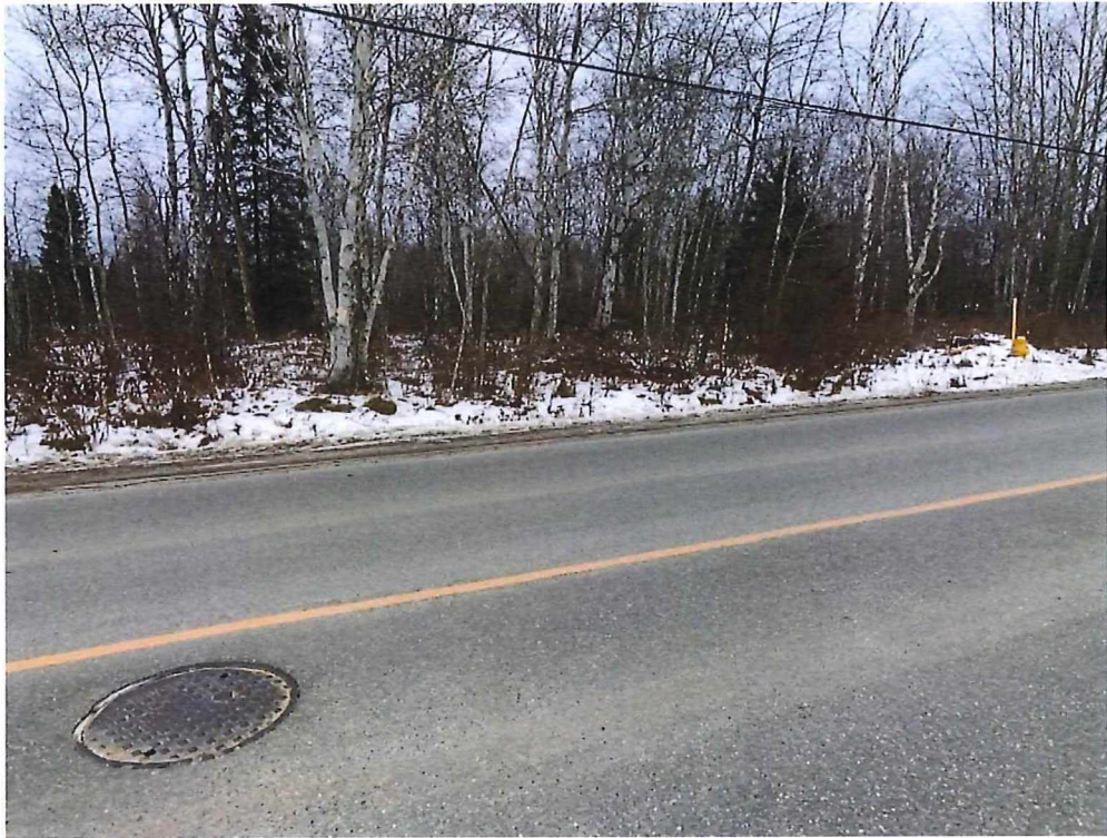
Figure 7: View of the subject property's public road frontage, existing man-hole & fire hydrant
