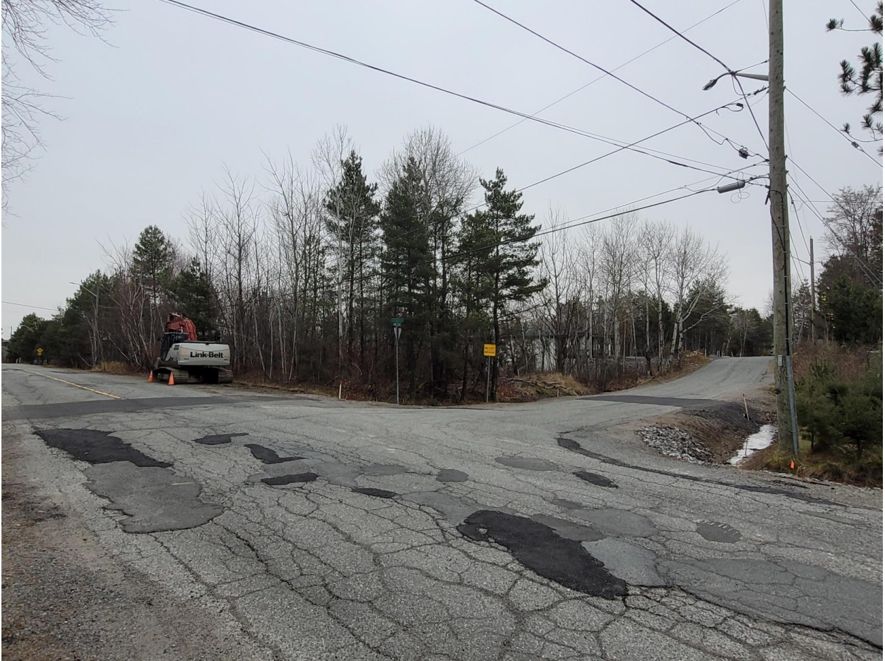
Photo 1: 1434 Gennings Street, Sudbury
