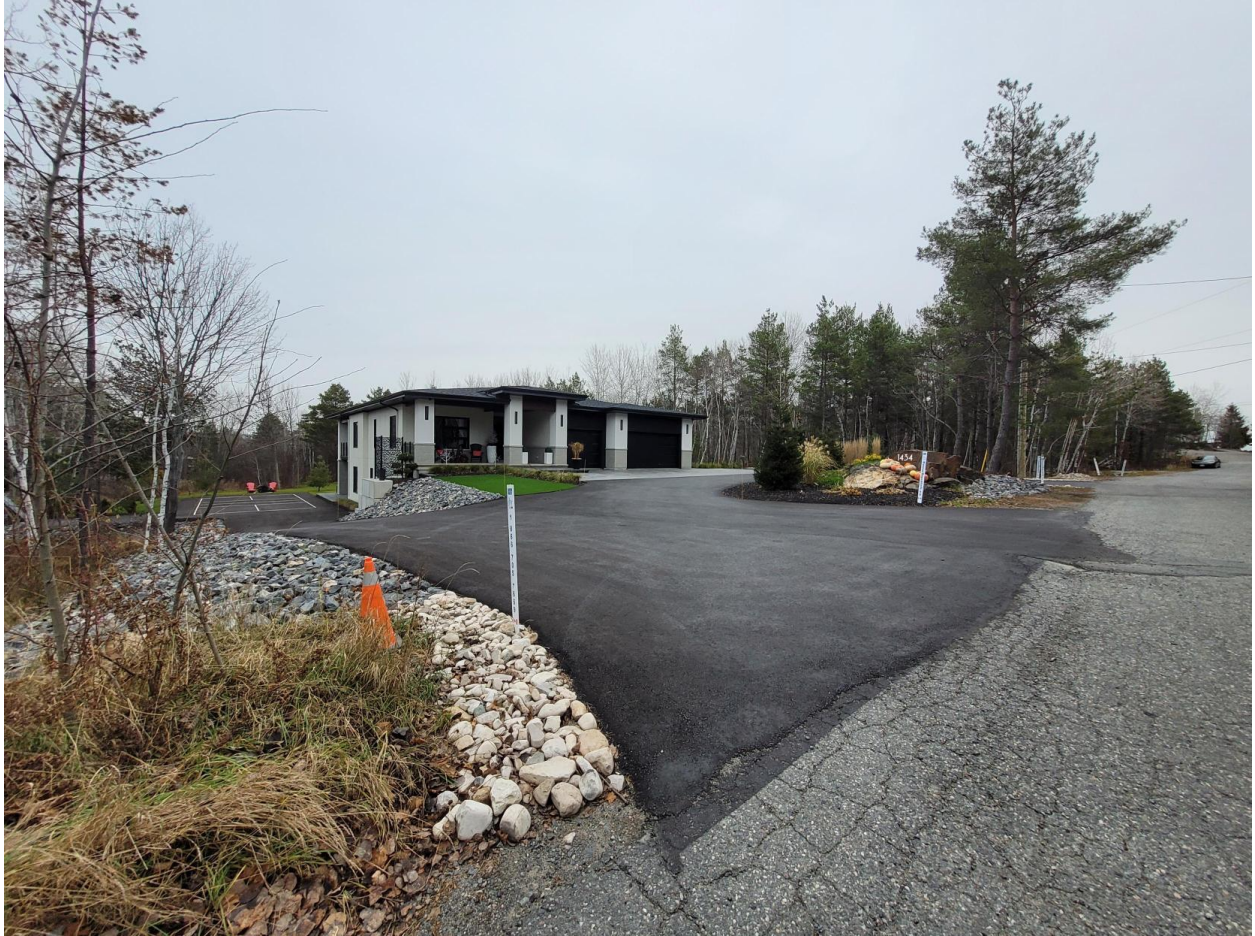
Photo 2: 1434 Gennings Street, Sudbury
