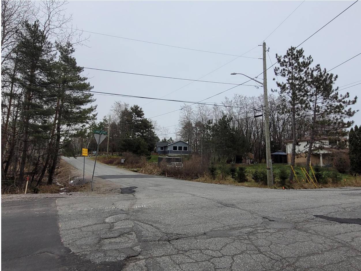
Photo 8: 1434 Gennings Street, Sudbury
