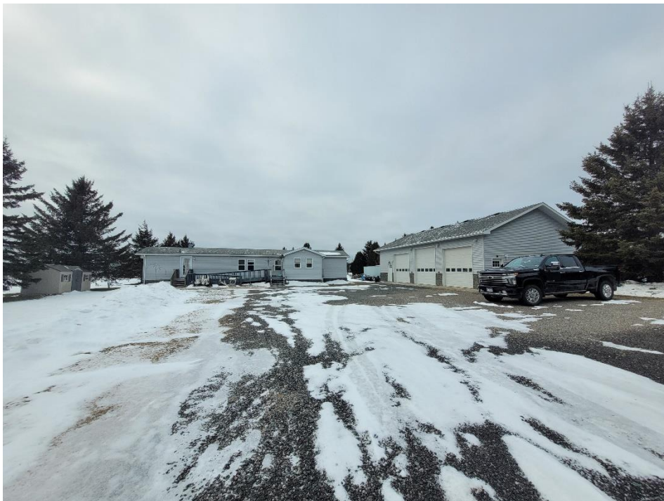
Photo 2: 754 Montée Principale, Chelmsford View of the garden suite (mobile home) and detached garage File 751-5/24-09 Photography: January 6, 2025
