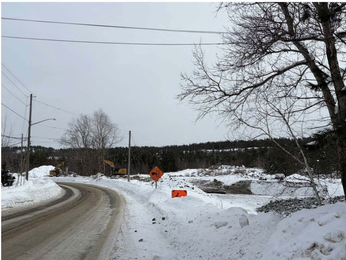
Photo 2: Frontage along Algonquin Road. File PL-RZN-2025-00040 Photography: January 30, 2026.
