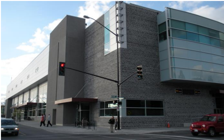
Figure 25 Rogers K-Rock Centre, Kingston ON (2008)
