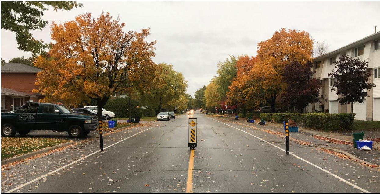
Figure 1: Temporary Traffic Calming Bollards Installed on Auger Avenue
