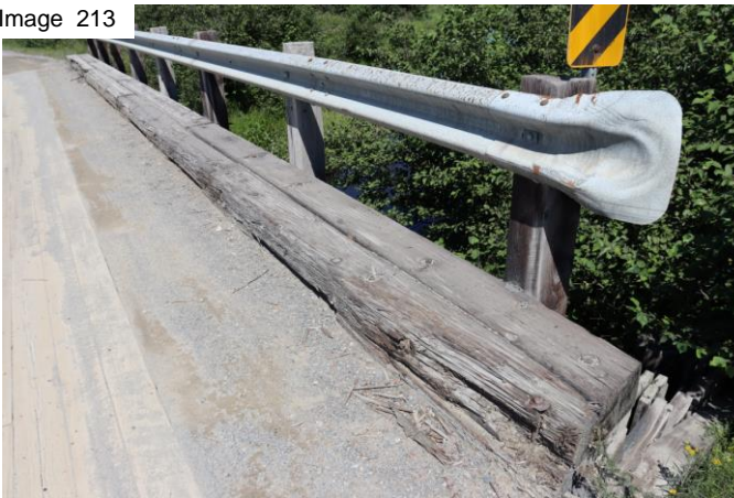
South deck surface damaged boards
