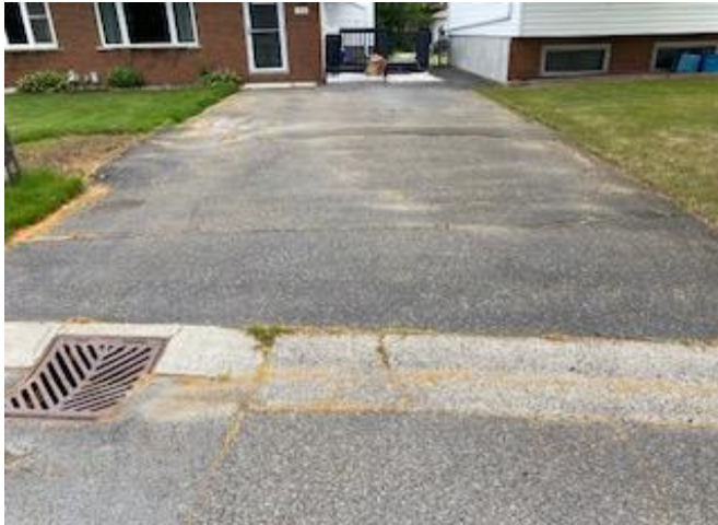
Figure 4a – Driveway at 1858 Huntington Drive
