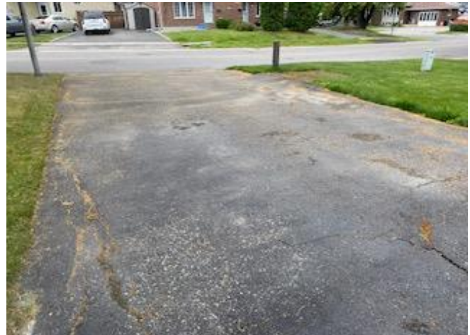
Figure 4b – Driveway at 1858 Huntington Drive
