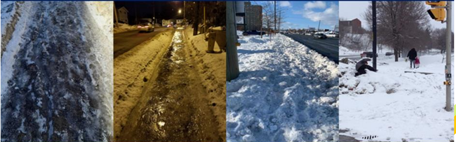
Icy, uneven surfaces make sidewalks impassable. Water on ice is especially treacherous.
