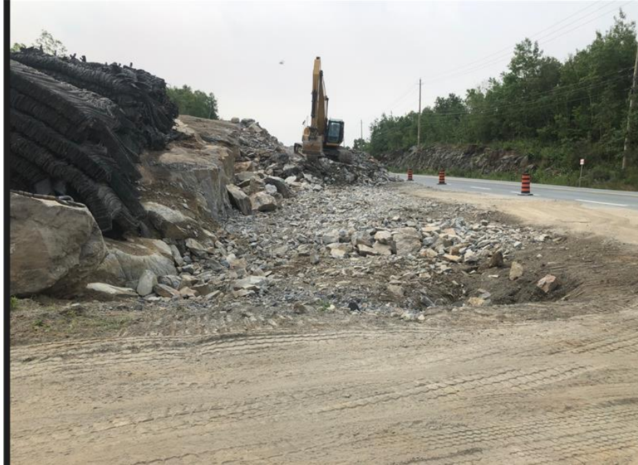
Figure 14: Long Lake Road - Rock removal from clear zone
