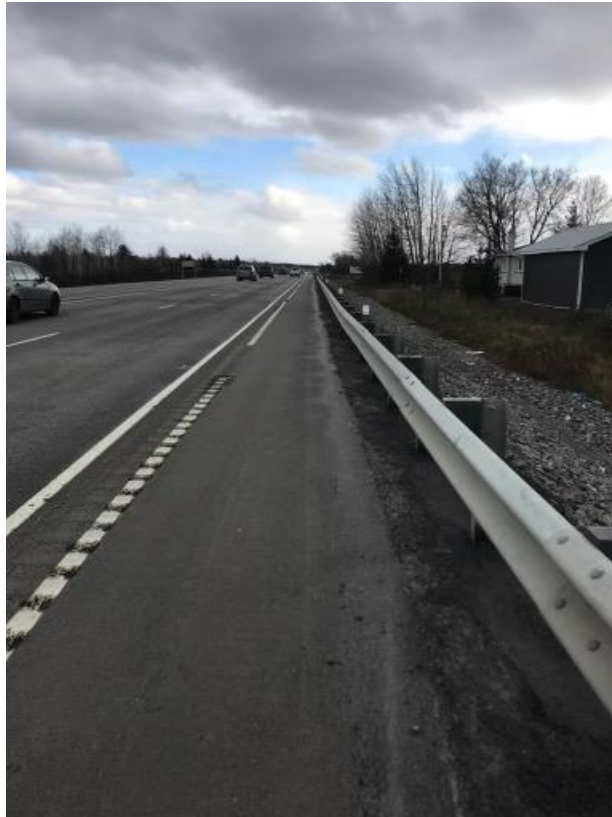
Figure 133: M.R. 35 - Paved Shoulder, Guiderail and Rumble Strip
