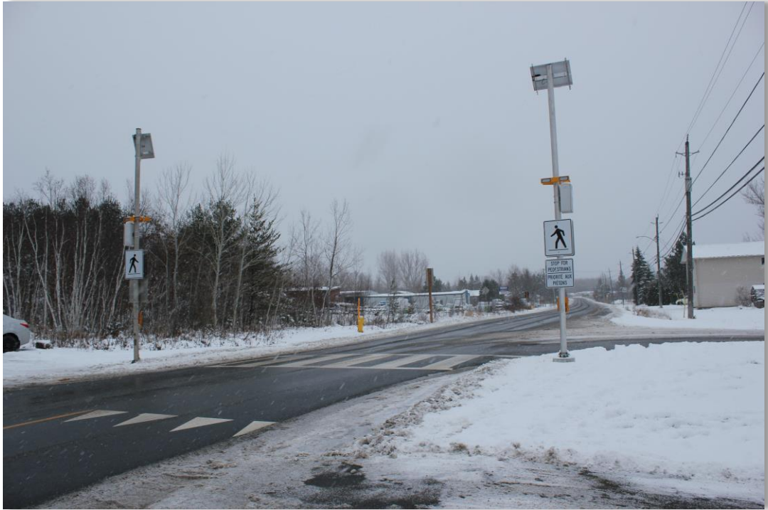
Figure 9: Type C Pedestrian Crossover on Hill Street in Wahnapiatae
