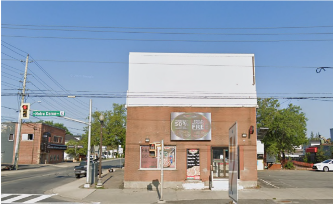
Pre-improvement Façade 497-509 Notre Dame Ave
