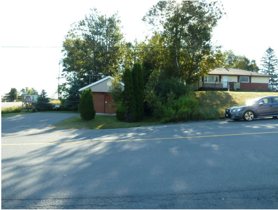
Photo 5: Centennial Drive, Hanmer Water booster station and single detached dwelling on Centennial Drive File 751-7/22-008 Photography: August 17, 2022
