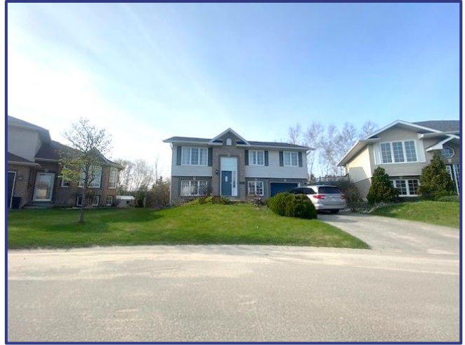
Figure 5: Single Detached Dwellings along Vintage Way east of Subject Lands
