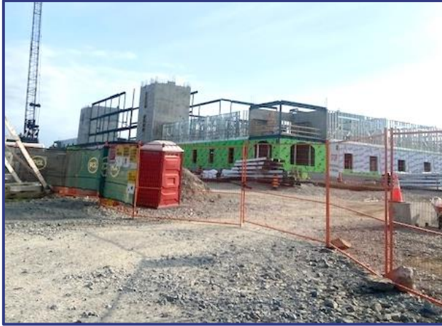
Figure 8: Long Term Care Home under construction on Algonquin Road
