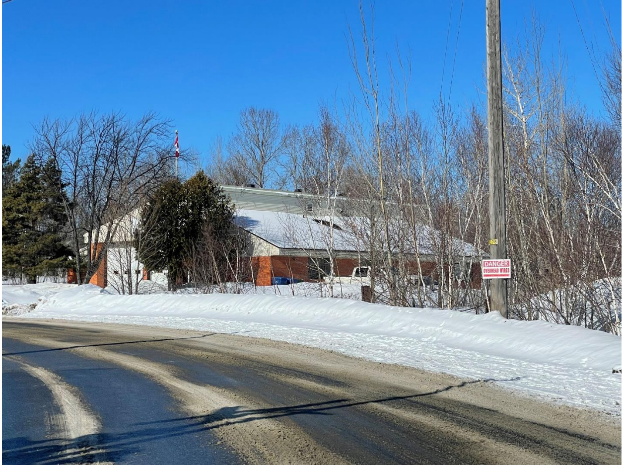
PHOTO #4 – Existing fire station building (ie. Minnow Lake Fire Station) situated to the immediate west of the southerly-most portion of the subject lands as viewed from Second Avenue looking north.
