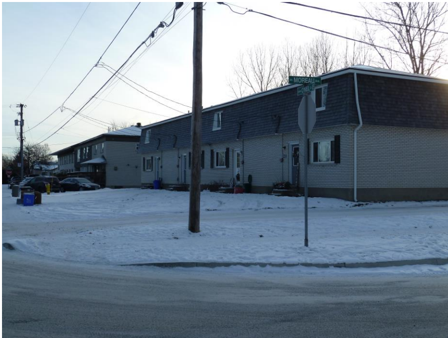
Photo 2: 223, 227, 231 & 235 O'Neil Drive East, Garson Four-unit row dwelling to be consolidated with 219 O'Neil Drive East Files 751-3/22-003 & 701-3/22-002 Photography: December 14, 2022
