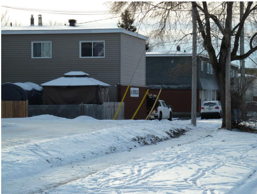
Photo 6: 40 Moreau Avenue, Garson 50-unit row dwelling complex located south of subject lands Files 751-3/22-003 & 701-3/22-002 Photography: December 14, 2022
