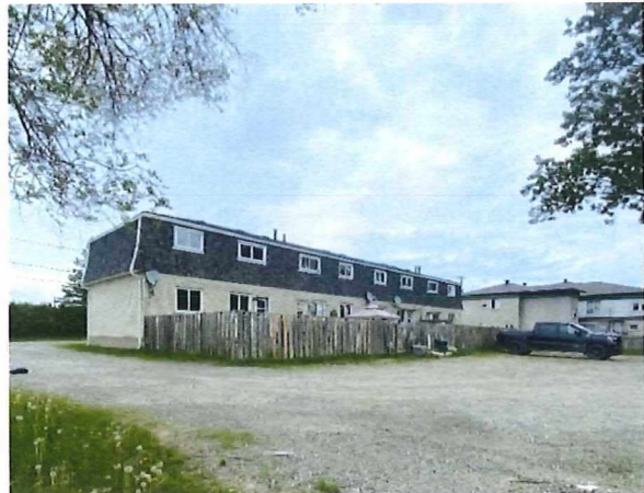
Figure 8: View of 223-235 O'Neil Drive E from Moreau Avenue
