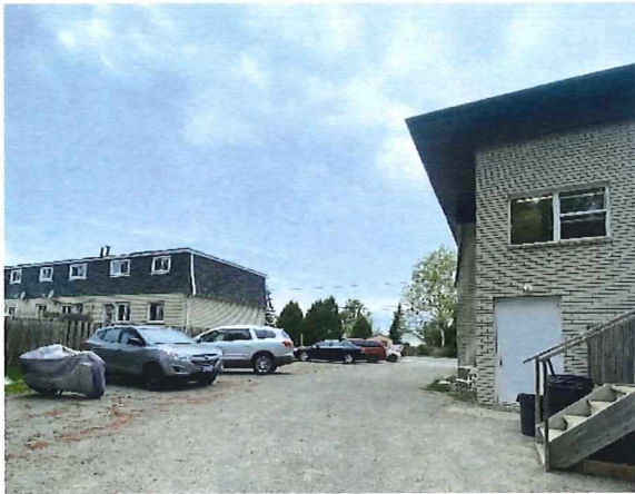
Figure 7: Westerly Interior Side Yard of 219 O'Neil Drive E facing 223-235 O'Neil Drive E
