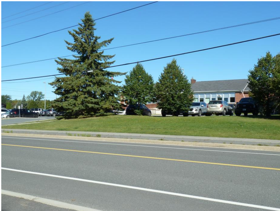
Photo 8: 2650 Algonquin Road, Sudbury Algonquin Road Public School located north of subject land File 751-6/22-009 Photography: September 29, 2022
