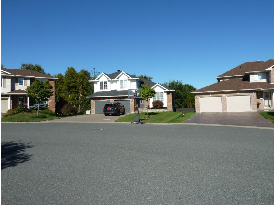
Photo 11: 50 Cognac Court, Sudbury Single detached dwelling on Cognac Court directly abutting easterly limit of subject land File 751-6/22-009 Photography: September 29, 2022
