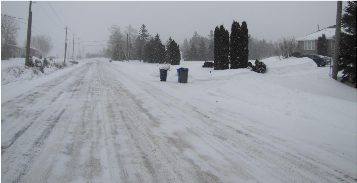
Photo 2. Bruno Street and surrounding rural residential uses, viewed looking east from the subject lands. Photo taken February 23, 2023, CGS File 751-5/23-01.
