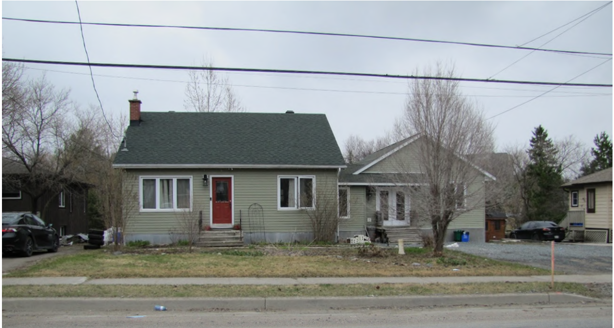
Photo 1. Subject lands, 1258 Southview Drive, facing southeast. Photo taken April 17, 2023. CGS File 751-6/23-02.
