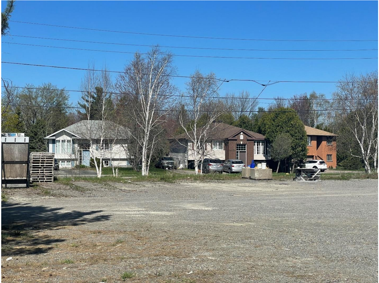
PHOTO 4: 2123-2177 Long Lake Road & 250 St. Charles Lake Road, Sudbury Existing low density residential dwellings to the immediate west of the subject lands having frontage on Brenda Drive File 751-6/22-21 (Photo Date: May 11, 2023).
