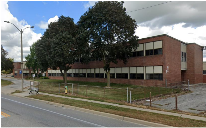
Figure 6 – Former Leamington District Secondary School
