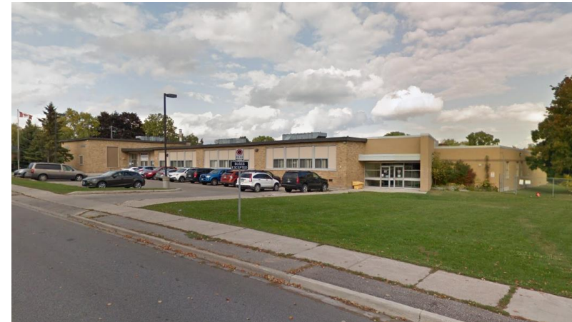
Figure 25 - Former Bradford Public School
