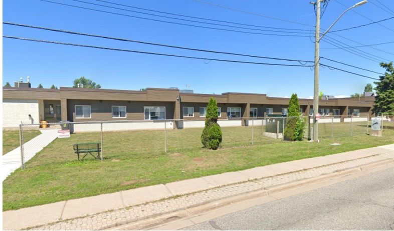
Figure 27 – Homeward Bound Housing Complex (after renovation)
