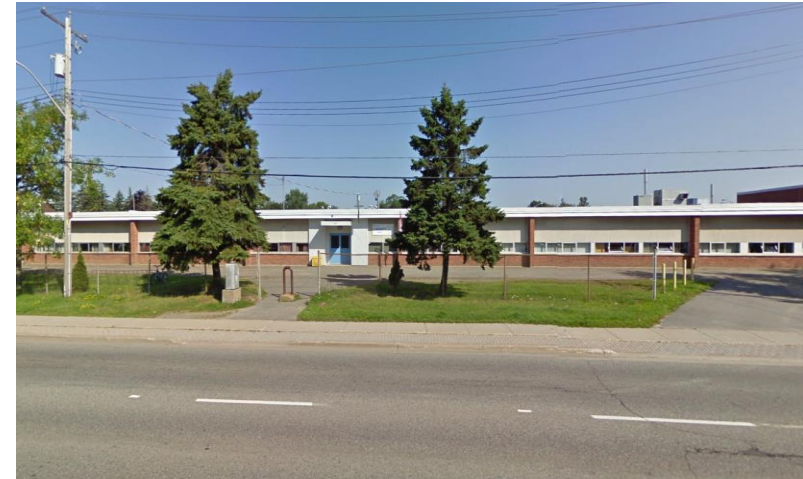
Figure 26 - Former St. Bernadette Catholic School (before renovation)
