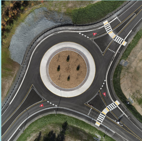
Completed a new roundabout in Falconbridge at the intersection of Longyear Drive and Edison Road, retiring and regreening an 800-metre section of Longyear Drive.
