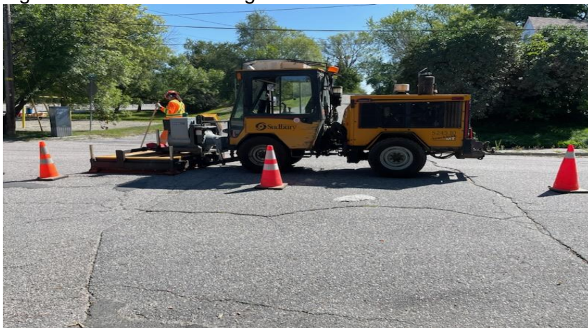
Figure 5 – Infrared Patching in Summer
