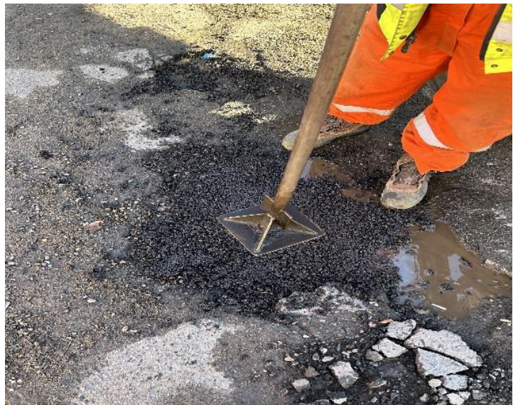
Figure 3b – Patching in a Wet Environments
