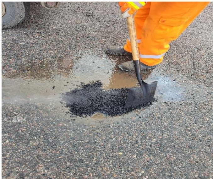
Figure 3a – Patching in a Wet Environments
