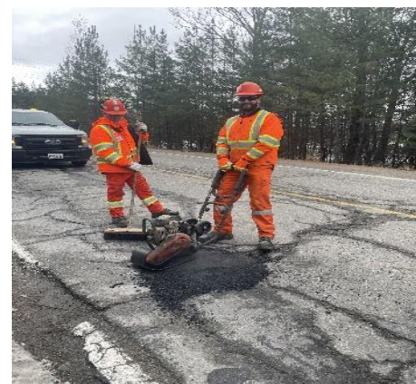
Figure 10b – Plate Tamper
