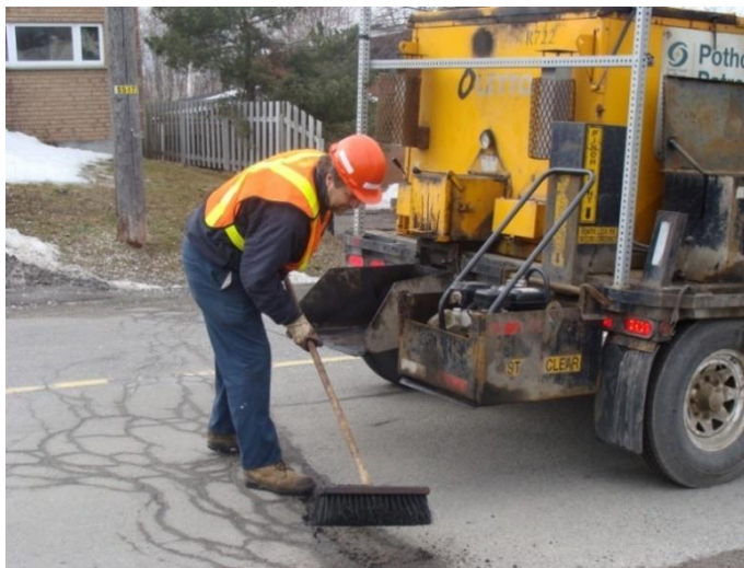
Figure 2a – Clean Pothole with Broom
