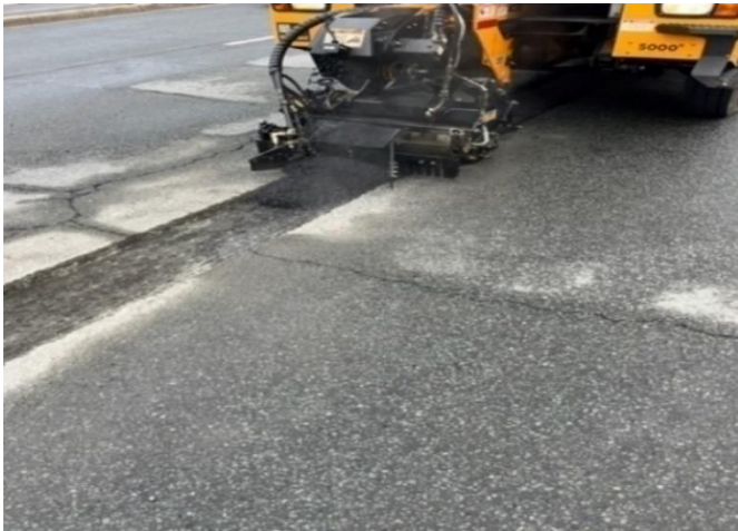
Figure 11a – Paving behind “Small Grinder” Crew
