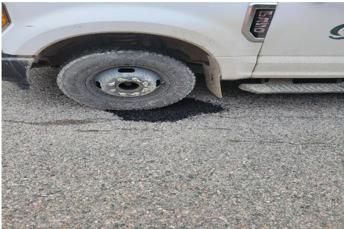
Figure 4a – Throw and Roll Patching
