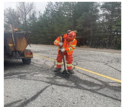
Figure 10c – Hand Tamper
