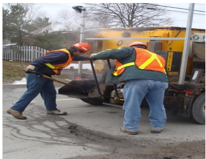
Figure 2b – Unload Patching Material from Hot Box
