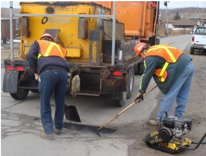
Figure 2c – Place and Shape Material
