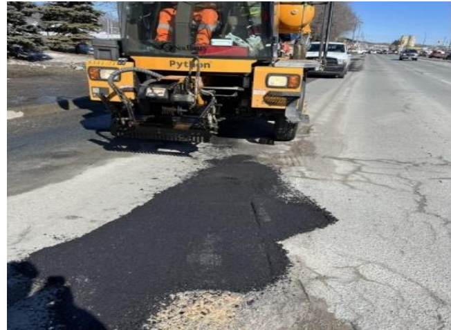
Figure 11b – Asphalt Overlay
