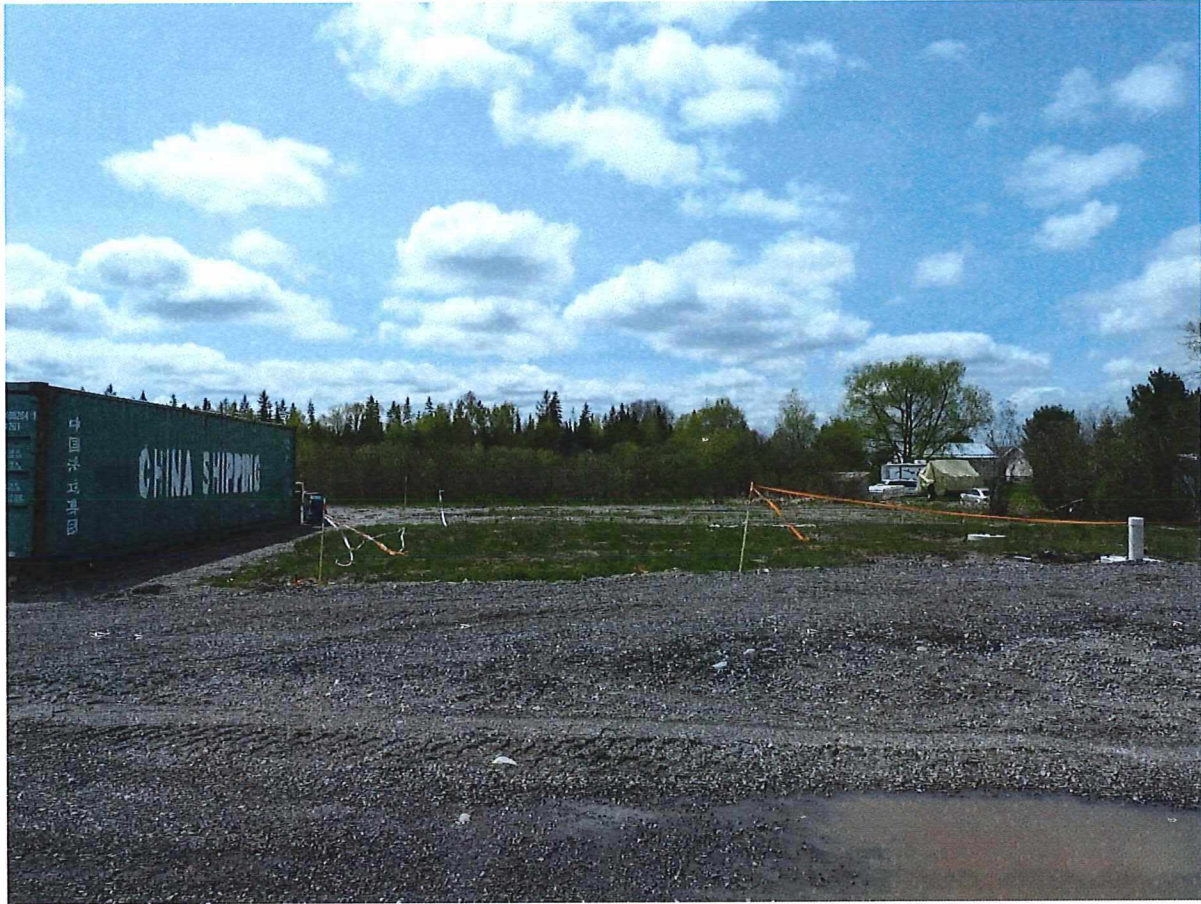
Photo 3: Joanette Road, Chelmsford Location of septic field bed behind main building with shipping containers at left Files 701-5/19-1 & 751-5/19-2
