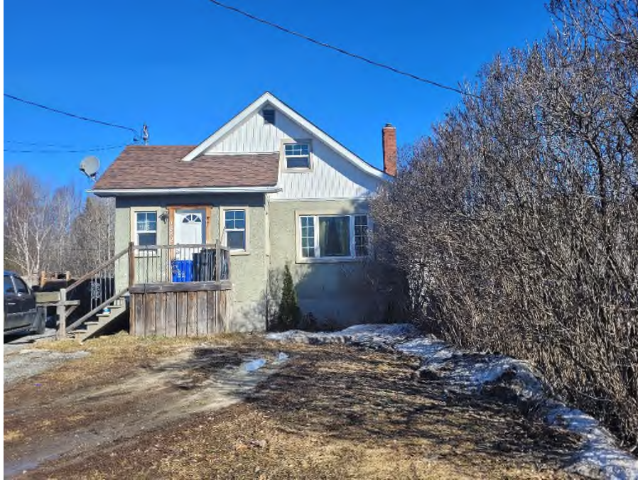
Photo 5: 1876, 1882 & 1890 Bancroft Drive, Sudbury
