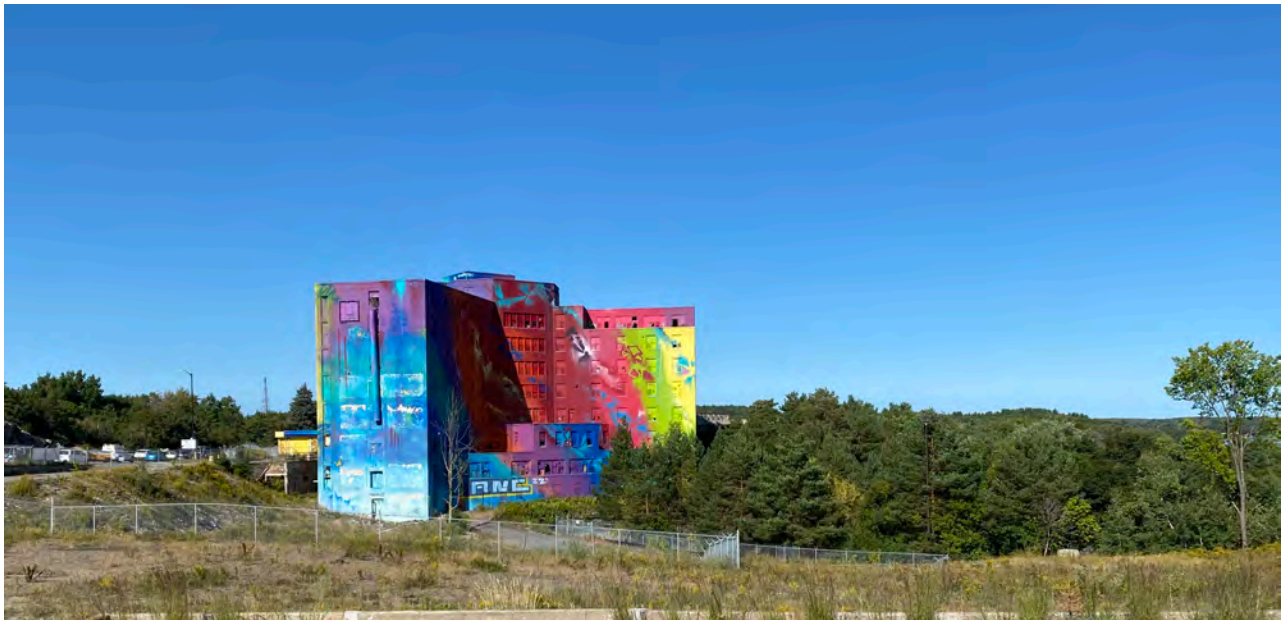
700 Paris Street existing site, looking north from adjacent parking lot
