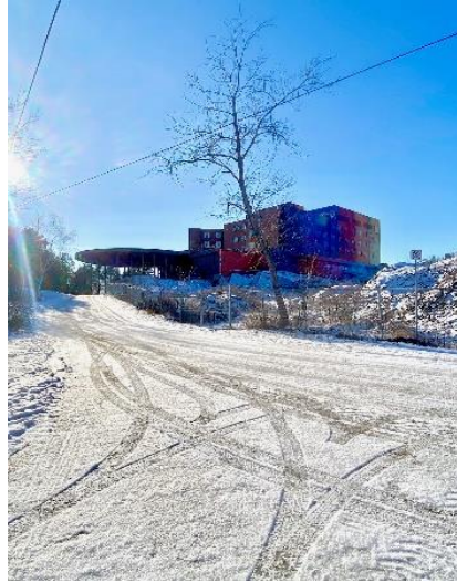
Figure 6: View of Subject Lands from Bell Park Road
