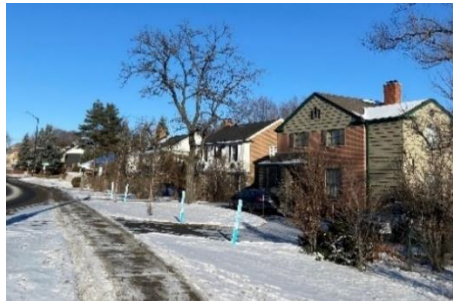
Figure 15: View of single detached dwellings north of subject lands (East side of Paris Street)
