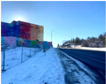
Figure 8: View of existing building looking south along Paris Street
