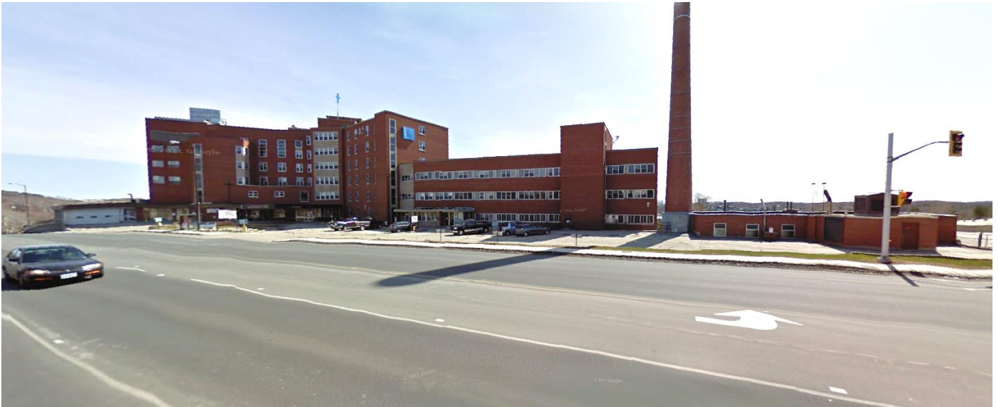
Figure 3: View of the former St. Joseph's Hospital from Paris Street (Image: Google Maps, August 2012).
