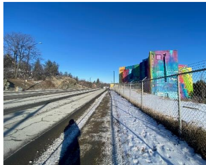
Figure 9: View of existing building looking North along Paris Street
