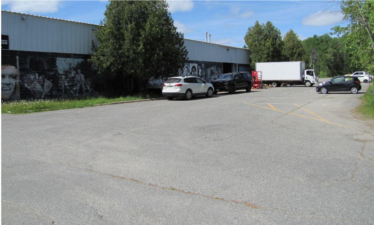
Photo 2. Subject lands, 828 Beatrice, facing northwest, showing the existing arena building and parking area. Photo taken May 24, 2024. CGS File 751-6/24-09.
