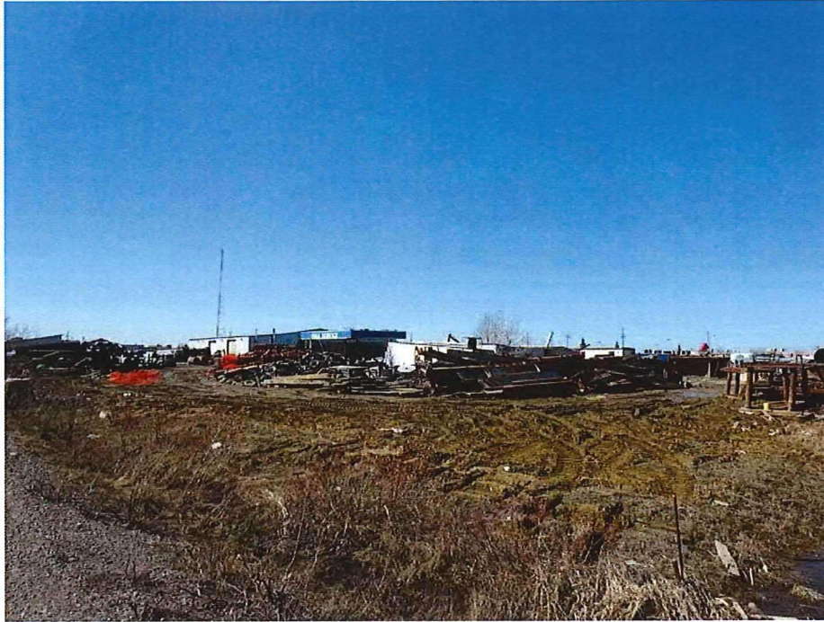
PHOTO 3 SUBJECT LANDS VIEWED LOOKING SOUTH WEST FROM THE NORTH WEST CORNER OF THE SITE FROM RADISSON AVENUE
