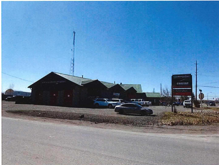
PHOTO 4 3248 RADISSON AVENUE, SOUTH OF THE SUBJECT LANDS, VIEWED LOOKING SOUTH EAST FROM MUNICIPAL ROAD 15 AND RADISSON AVENUE
