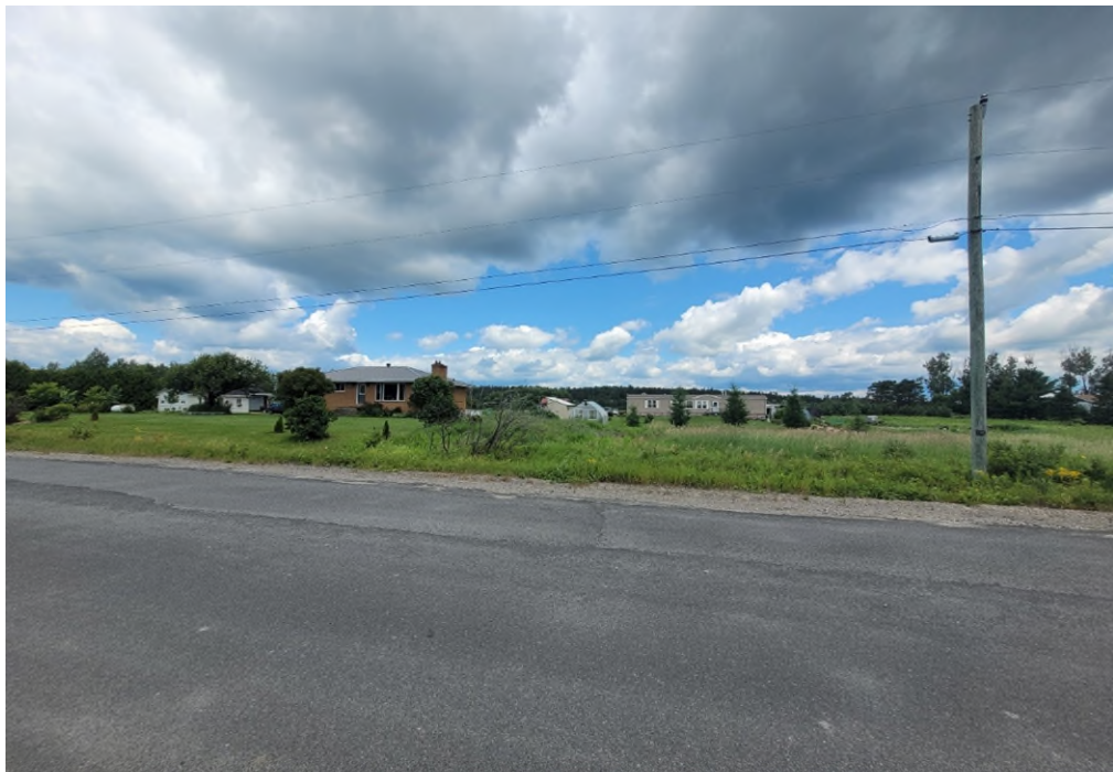
Photo 2: 2548 McKenzie Road, Chemsford. View of the subject parcel from McKenzie Road. The principal dwelling is the brick structure. The garden suite is to the right of the principal dwelling. File 751-5/24-04 Photography: July 9, 2024
