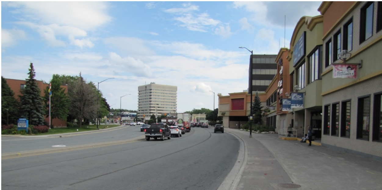
Photo 6. Subject lands at 40 Elm Street showing the east side of the existing building along Notre Dame Avenue, facing south. Photo taken July 8, 2024. CGS File 701-6/24-05 & 751-6/24-08.
