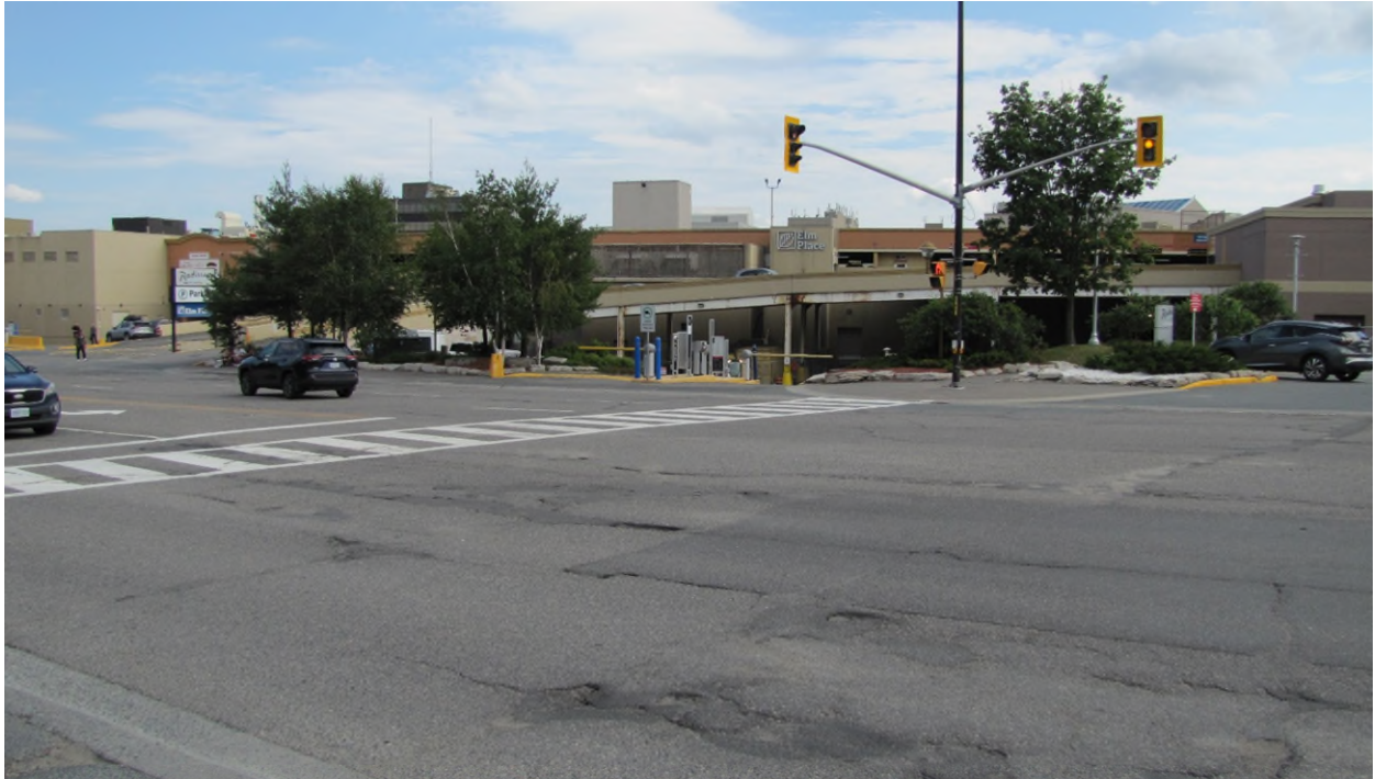
Photo 5. Subject lands at 40 Elm Street showing the north side of the existing building and the loading dock extending from Ste. Anne Road, facing south. Photo taken July 8, 2024. CGS File 701-6/24-05 & 751-6/24-08.
