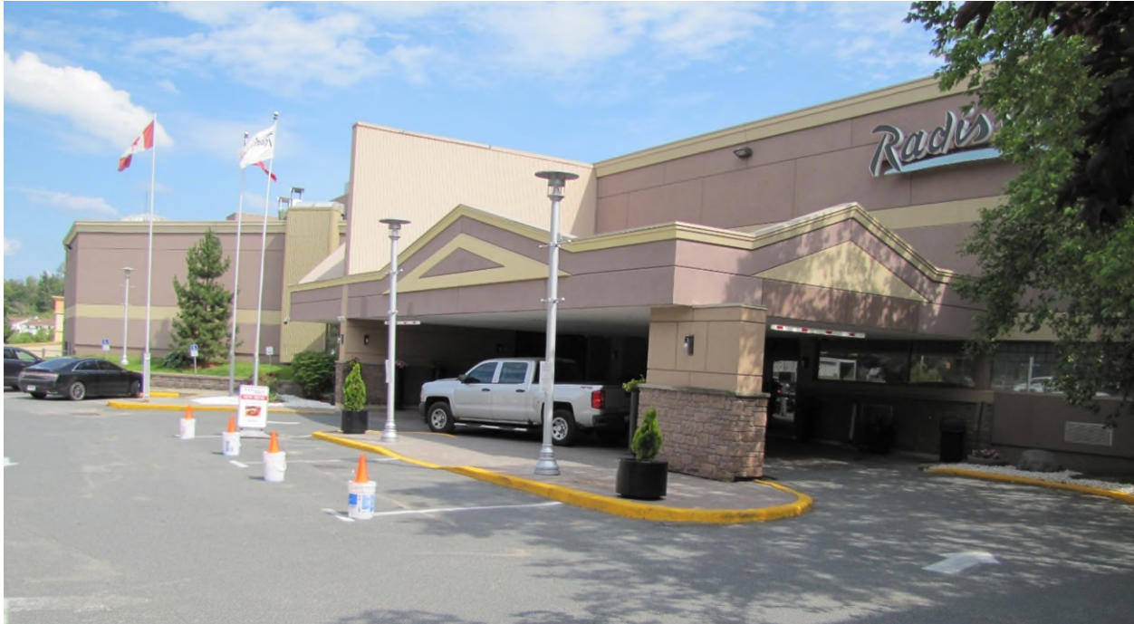
Photo 7. Adjacent hotel use to the northwest of the subject lands, facing east. Photo taken July 8, 2024. CGS File 701-6/24-05 & 751-6/24-08.
