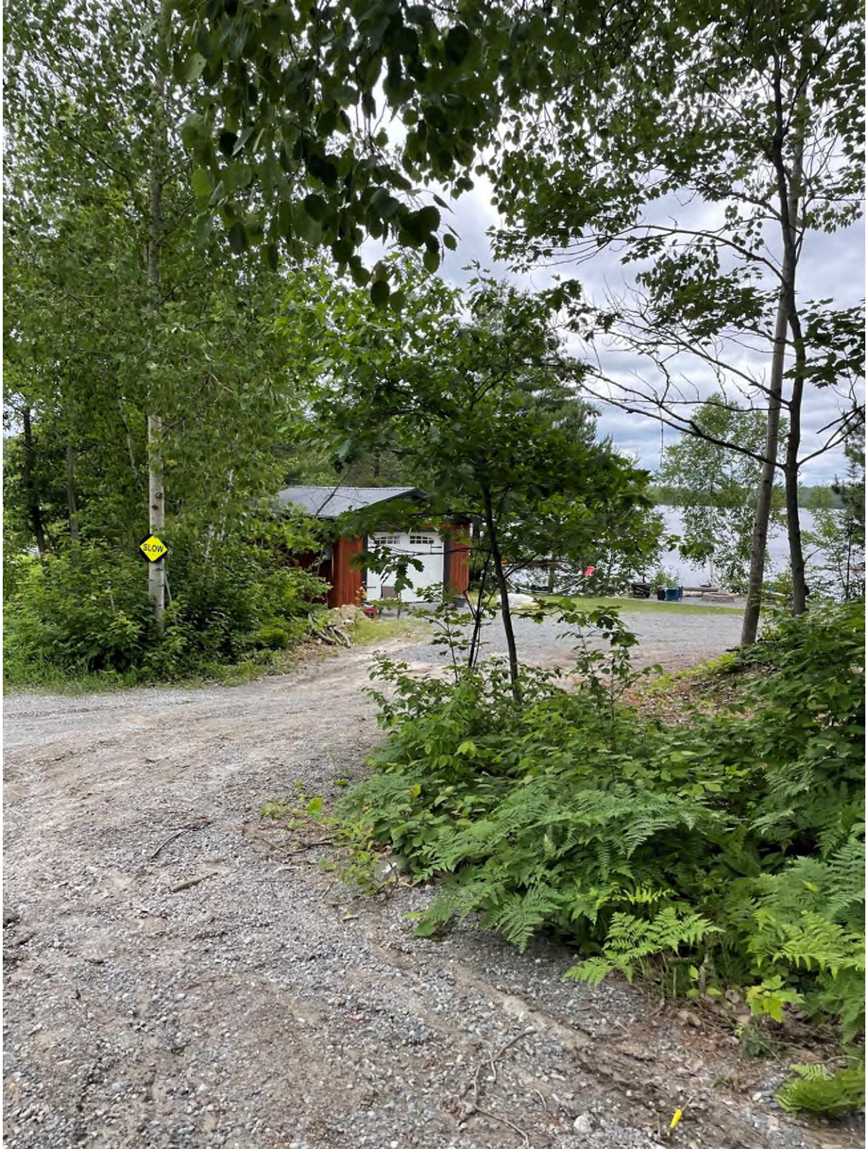
Photo 1. Existing driveway and accessory building. Photo taken June 30 th , 2024. CGS file 751-3/24-02.
