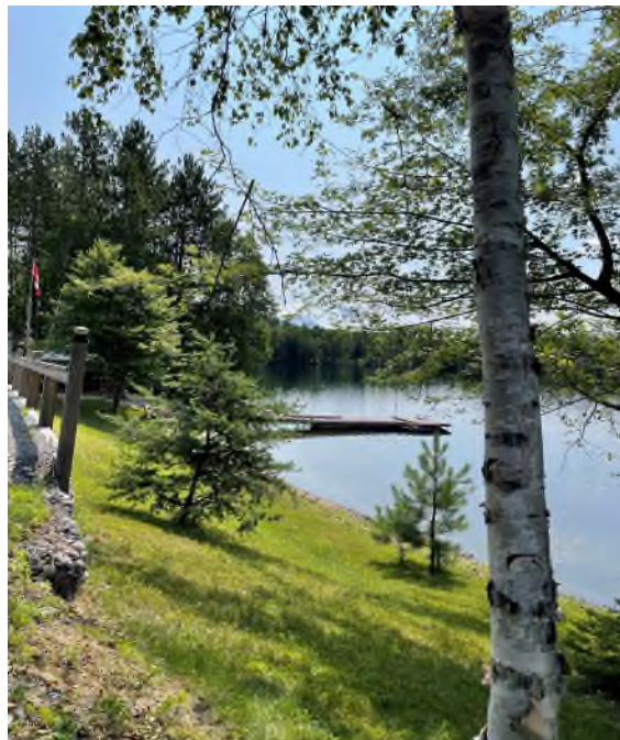
Photo 2. Grassed area and retaining wall on the subject lands, crown land abutting 3247 Hanmer Lake Road East. Photo taken July 22 nd , 2024. CGS file 751-7/24-05.
