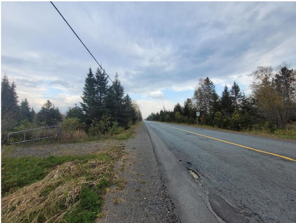
Photo 6: 0 Dominion Drive, Hanmer. View of the Dominion Drive looking west with the subject parcel to the left File 751-7/24-07 & 701-7/24-01 Photography: October 6, 2024
