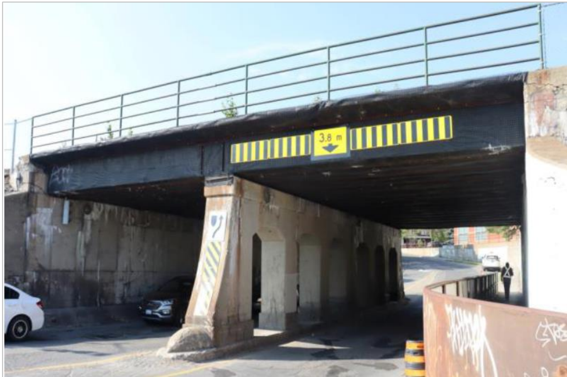
Figure 1. College Street Underpass, looking southbound (from 2022 Inspection Report)
