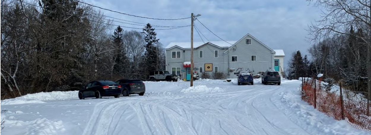
Photo 1. Subject lands at 58 Jacobson Drive, showing the existing building, facing east. Photo taken December 6, 2024. CGS File 751-8/24-03.
