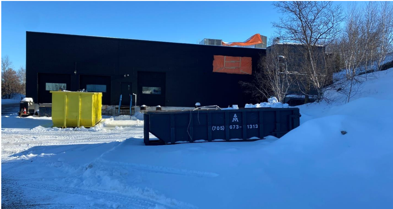
Photo 4. Subject lands at 363 York Street, showing the west side of the building, facing east, from the west side of the site. Photo taken December 13, 2024. CGS File 751-6/24-20.
