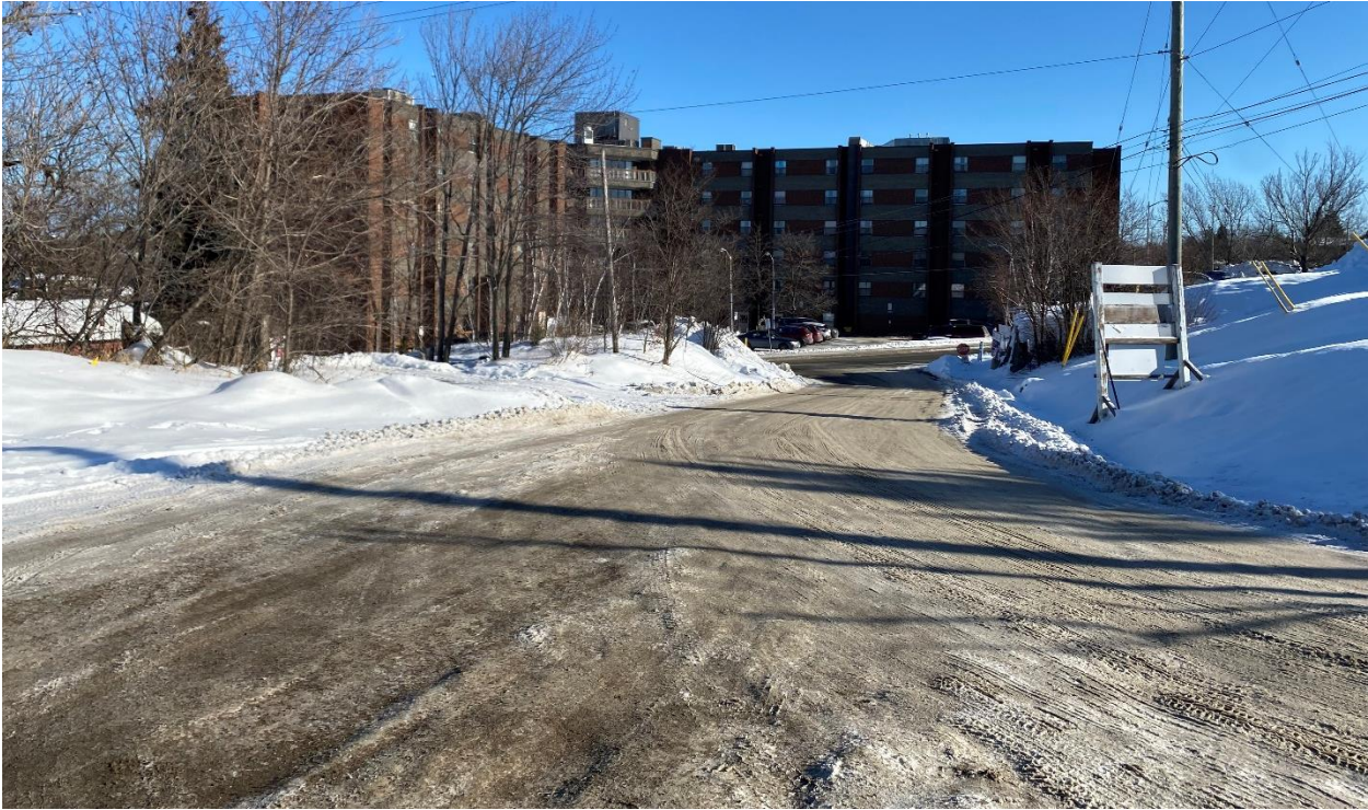
Photo 8. Health Sciences North Outpatient Centre to the east of the subject lands, facing east, from the access driveway to the subject lands. Photo taken December 13, 2024. CGS File 751-6/24-20.
