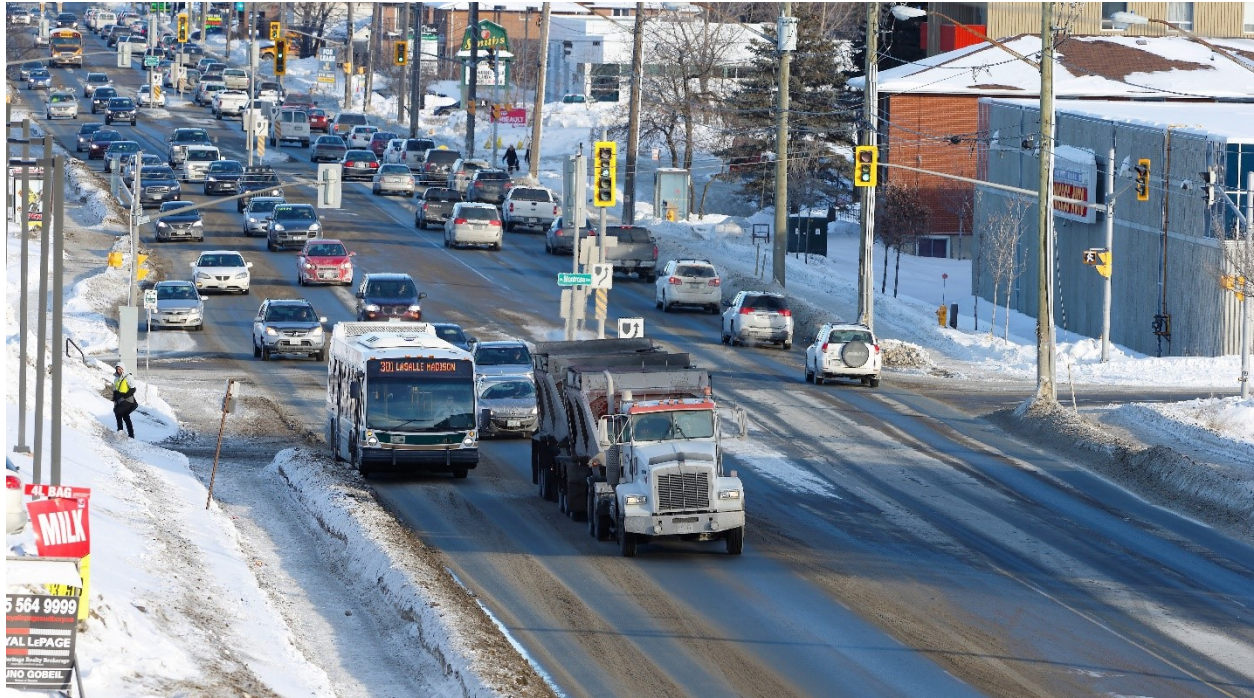
Figure 49. Example of lanes with snow storage
