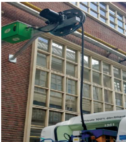
Figure 33. Example of Wall Mounted Cable Reel
