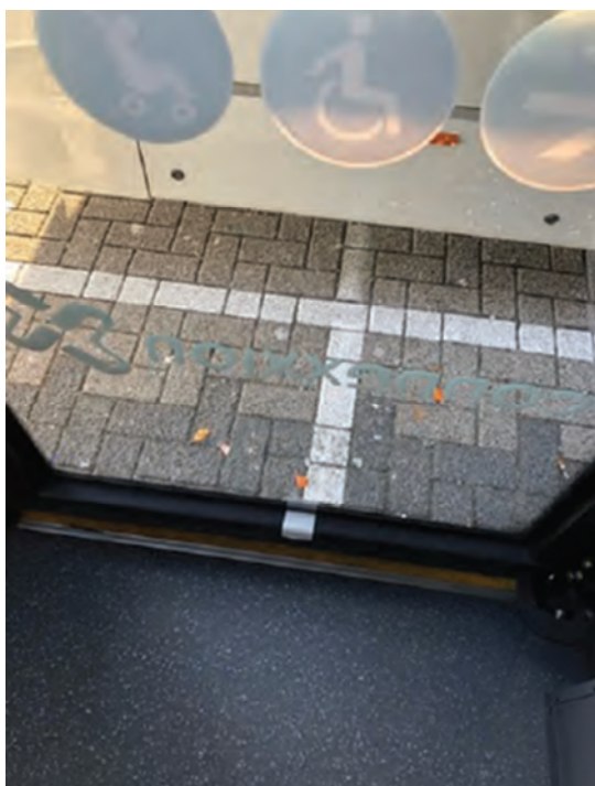
Figure 34. Example of Alignment Markers for Proper Bus Positioning 12
