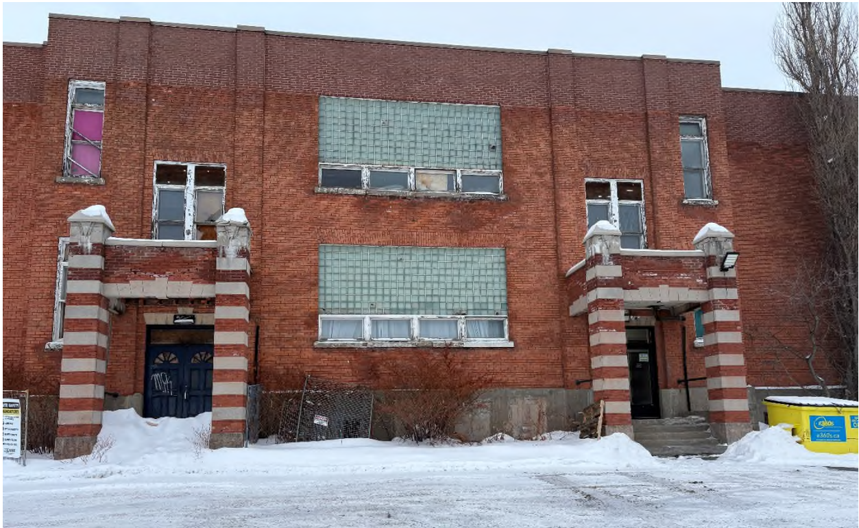
Photo 8. Existing building on the subject lands, facing north from the south side of the existing building. CGS Files PL-OPA-2025-00021 & PL-RZN-2025-00054). Photo taken February 26, 2026.
