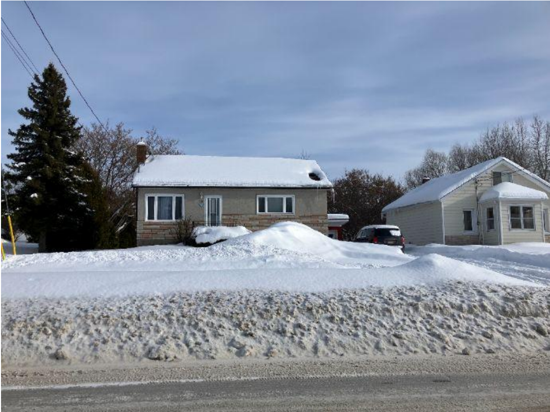
Figure 1: Existing residential dwelling, 62 Levesque Street (February 12, 2026)
