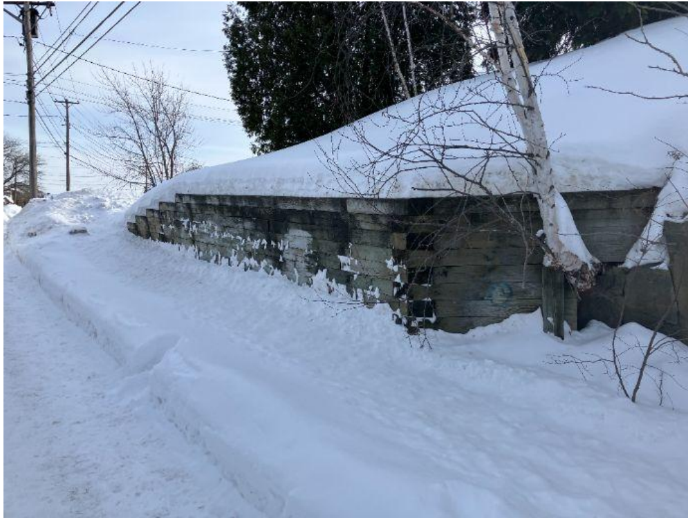
Figure 5: Existing retaining wall along Martindale Road (February 12, 2026)
