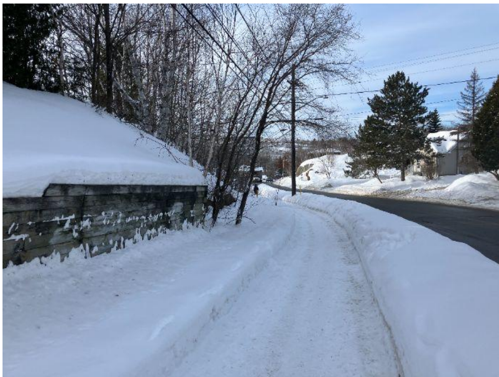
Figure 6: Retaining wall and sidewalk along Martindale Road (February 12, 2026)
