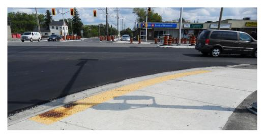
As part of the new Accessibility for Ontarians with Disabilities Act standards, tactile warning indicators are to be installed where an accessible walkway crosses a vehicle path. The purpose of the tactile warning indicators is to alert visually impaired pedestrians when they are approaching an intersection before they reach the curb ramp.
