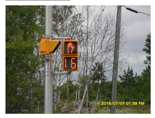
A common concern raised by pedestrians crossing intersections with traffic signals is the uncertainty of the time remaining to cross once the "Flashing Don't Walk" display begins. In response to this concern, the traffic signal industry developed the Pedestrian Countdown Signal (PCS) head. The PCS is an enhanced pedestrian signal head which displays the amount of time remaining to cross the intersection.
