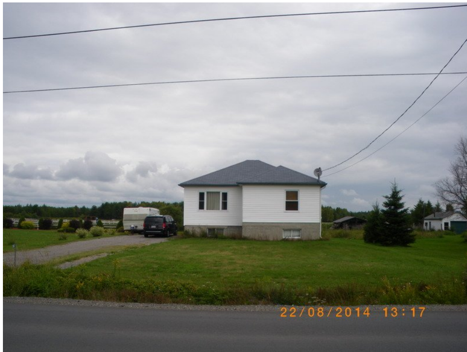
PHOTO 2 GARDEN SUITE ON SUBJECT LANDS, LOCATED WEST OF THE PRIMARY DWELLING, VIEWED LOOKING NORTH FROM GRAVEL DRIVE
