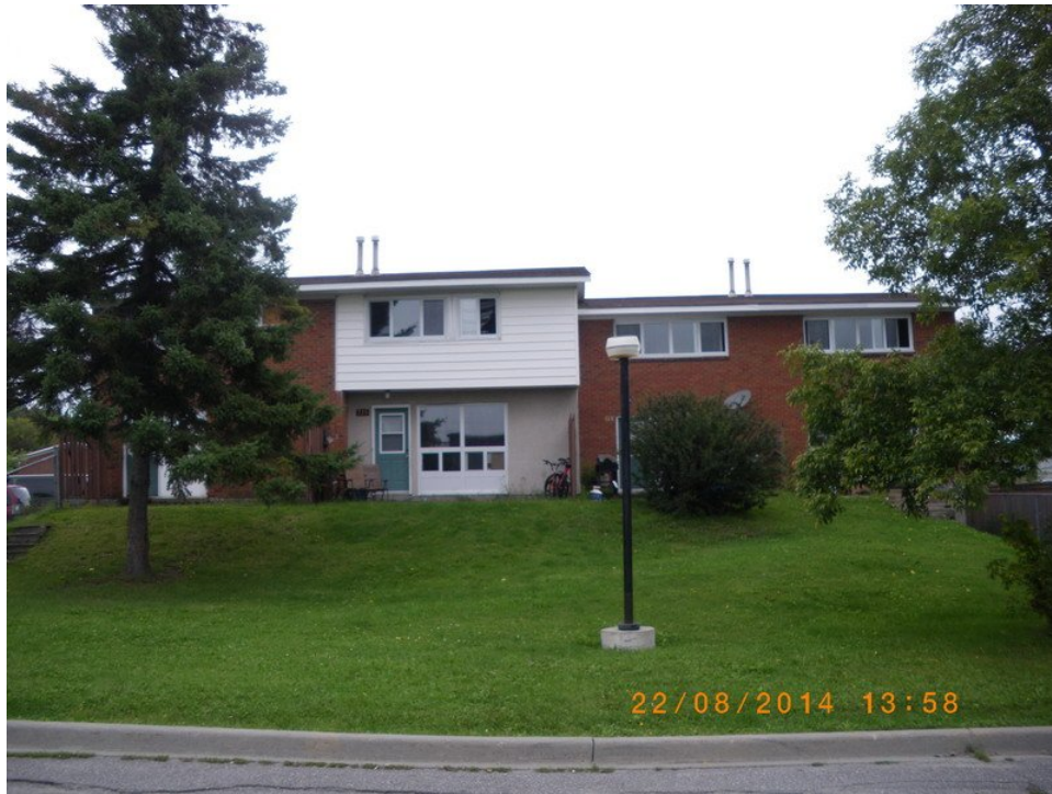
PHOTO 5 1200 LASALLE BLVD., NORTH OF THE SUBJECT LANDS VIEWED LOOKING NORTH FROM SPARKS STREET
